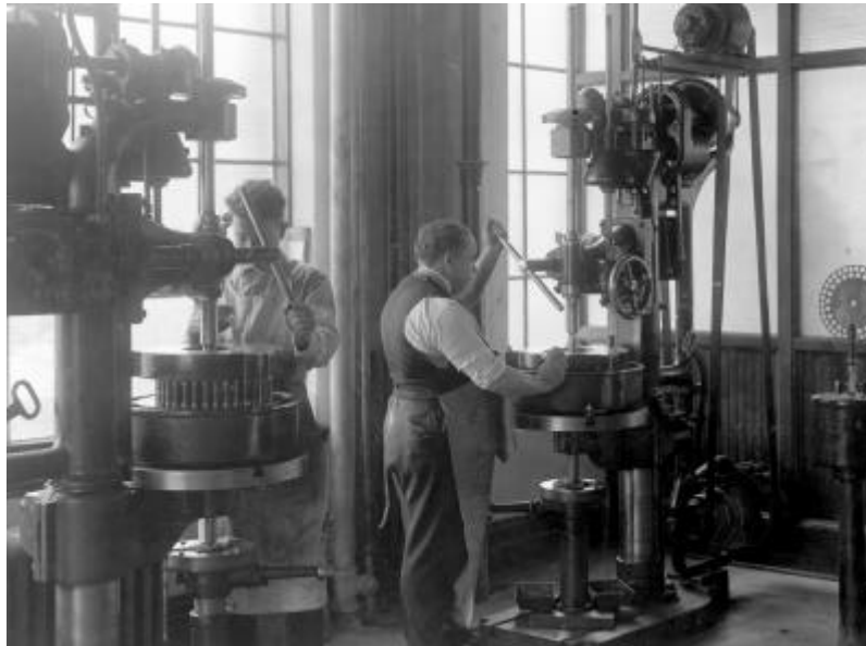
Figure 3. Precision gage blocks, manufactured at the Bureau in 1919, were lapped to exact nominal length.
